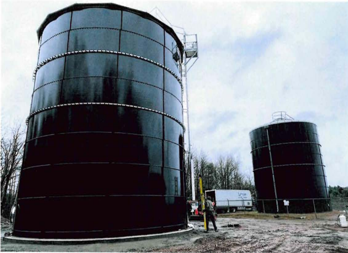
Redundant Potable Water Storage Tank at Human Service Complex
