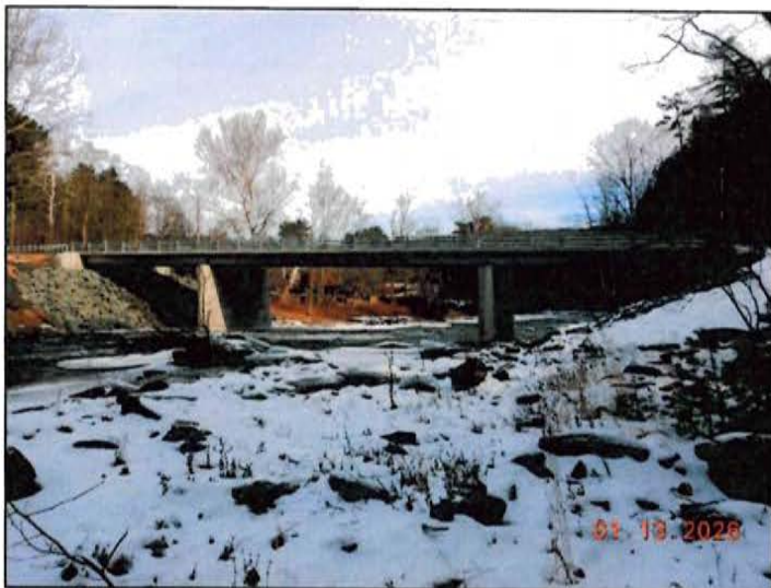
New County Bridge 82 on County Road 49/Oakland Valley Road in the town of Forestburgh. Typical example of successful procurement of 95% funding and contract administration.
