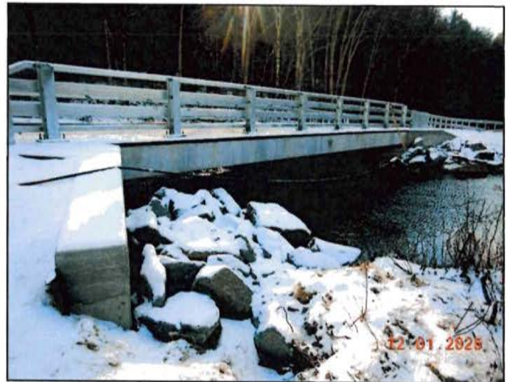
New County Bridge 270 on Flugertown Road, in the town of Neversink. Typical example of a bridge designed by the Division of Public Work's Engineering Bridge Unit and built by DPW's Bridge Operations Unit.
