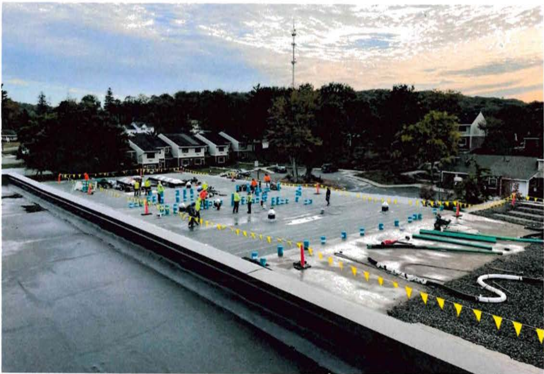
Government Center Annex Roof Replacement
