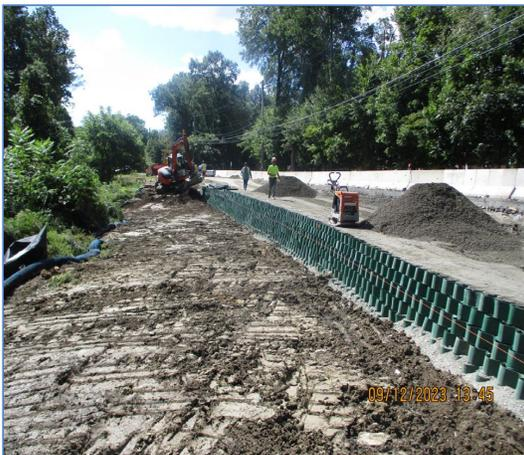
County Road 61 Embankment Repair—GRSS Geo-cell Retaining Wall
