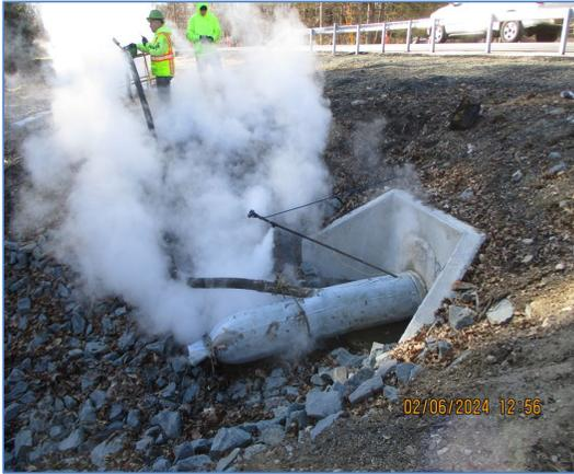
County Road 61 Drainage Repair—No Dig Cure-In-Place Slip Lining
